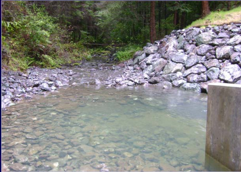
Roughened Riffle with Engineered Streambed Material Stabilizes Channel below Fishway
