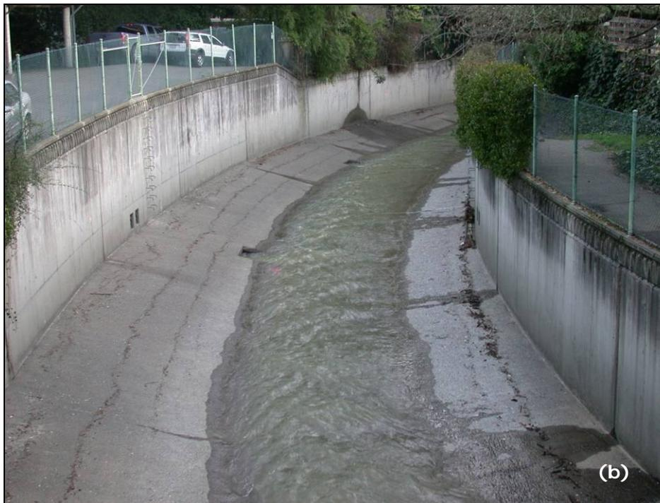
**Figure 1.3** – Dimensions of a typical straight channel reach (a) with v-shaped channel bottom and the channel bend downstream of the Kentfield Hospital Bridge (b) with the v-shaped bottom superelevated towards the outside of the bend.
