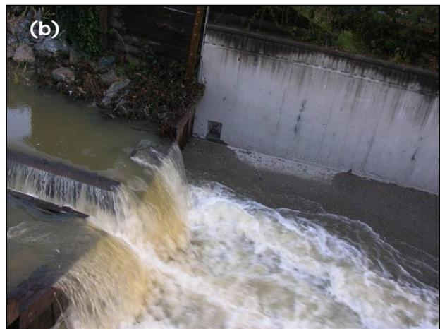
**Figure 1.5** - Existing Denil fish ladder and bypass weirs at the upstream end of Unit 3 (a) during low-flow in June 2005 and (b) at a typical steelhead migration flow in February 2007 following flood repairs.
