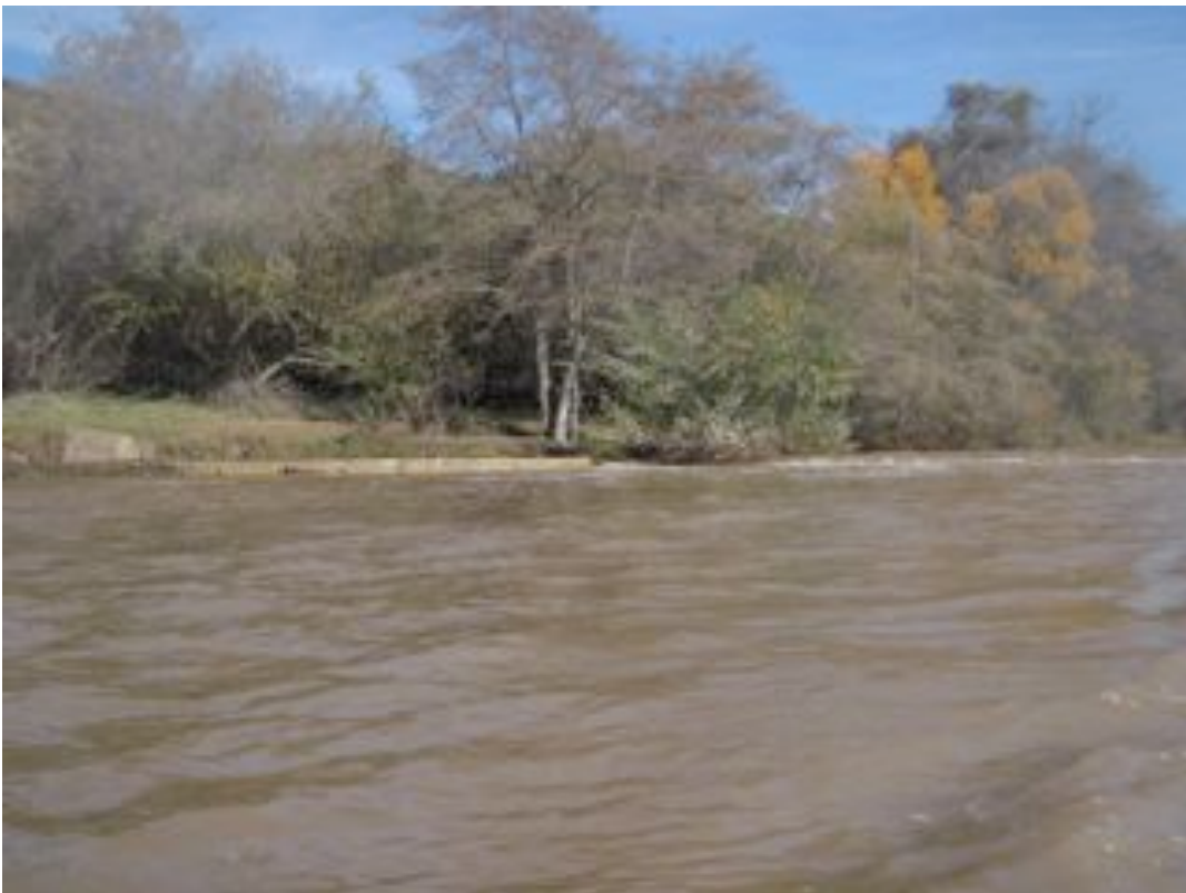
"Sisquoc" gage weir exposed at left (river-right) and submerge ~3/4 of channel width
