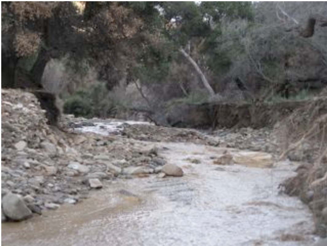
~ 800 ft. upstream of the former dam. Note downcutting of the channel into dam deposits
