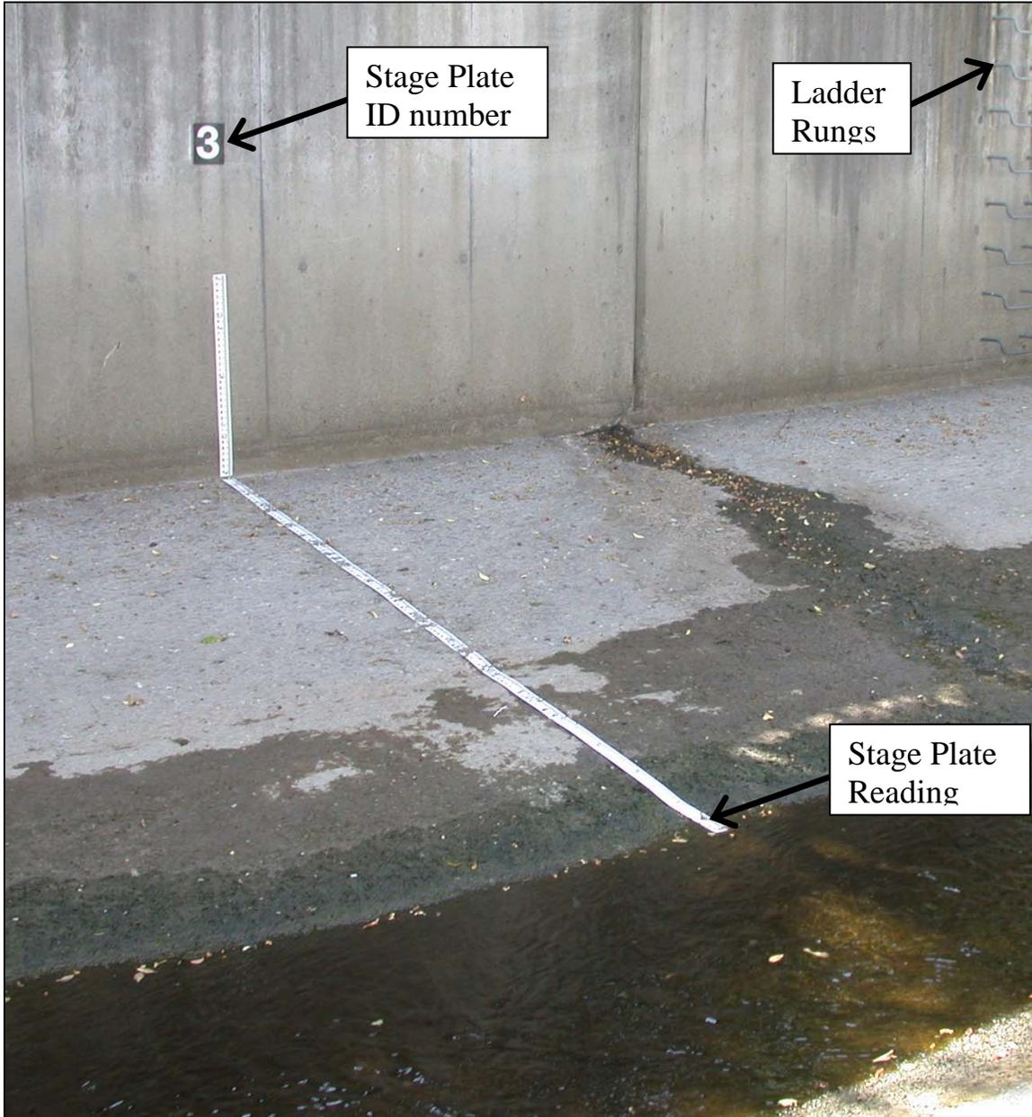
**Concrete channel showing the stage plate and the Stage Plate ID Number. Ladder rungs can be used to gauge water depth if the plate is fully submerged.**
