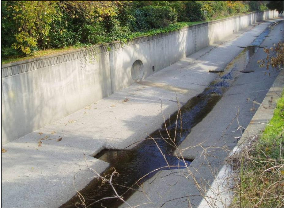
**Figure 1.4** – Upper section of Unit 3 with existing fish resting pools. Each pool is 4 feet long, 13 feet wide, and spaced 64 feet apart. The flat concrete bottom in each pool is approximately 0.1 feet below the channel invert.
