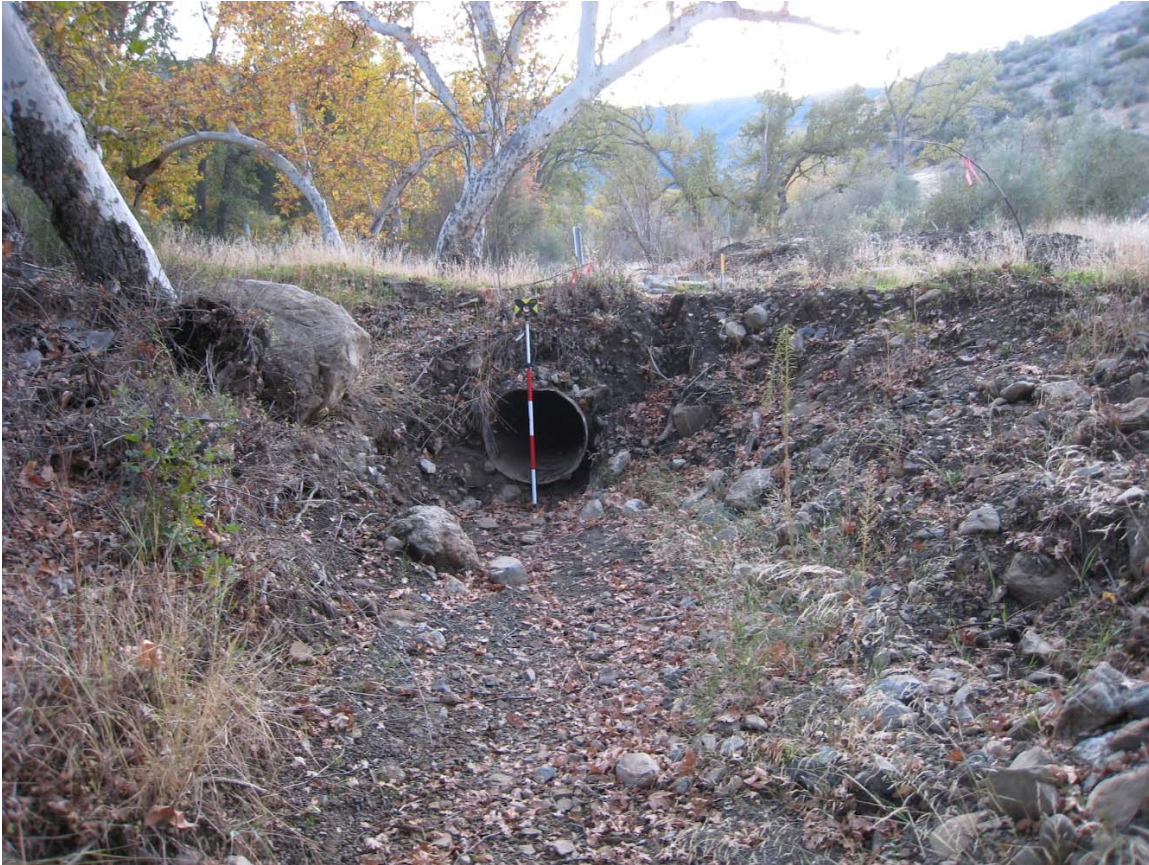
Figure 16 – Side channel culvert located approximately 125 -ft from the Upper Sunset Valley Road crossing. The culvert has a 3-ft diameter and is rusted, showing signs of regular sediment removal at the inlet. During high flows water diverted from the ford re-enter the channel at this location.
