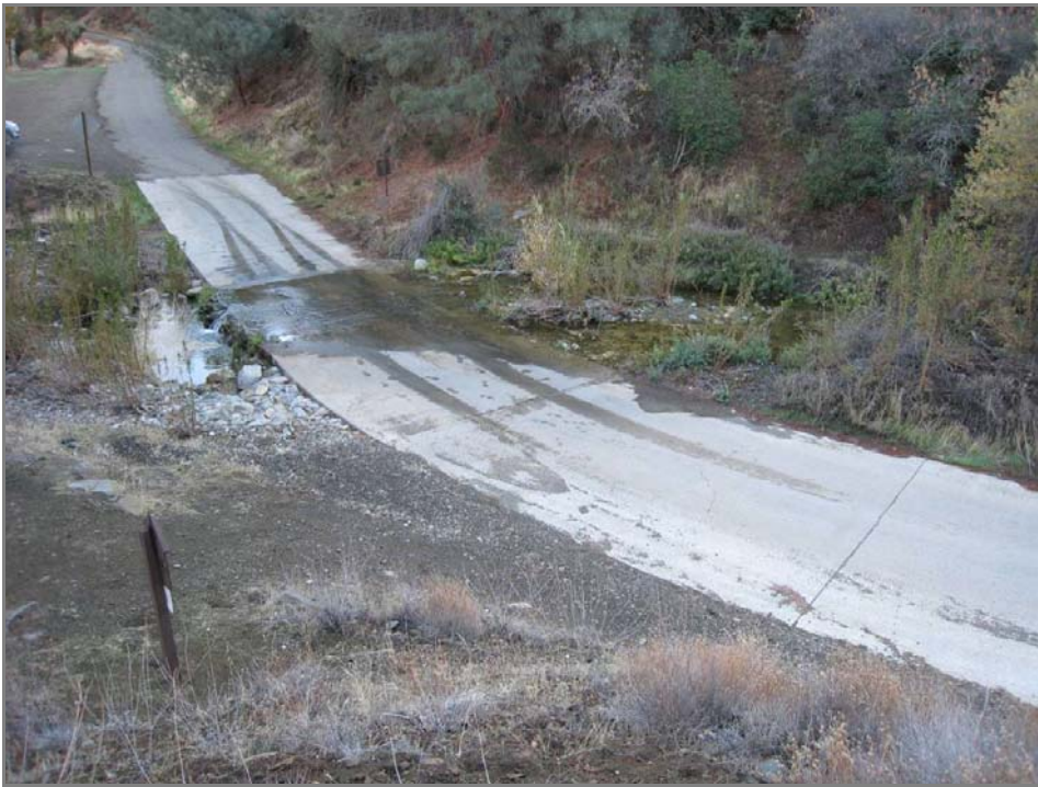
Figure 8 – Lower Sunset Valley Road at Davy Brown Creek (H-150'59-3). The 18-foot wide concrete low-water ford is located 130 feet upstream of the confluence with Manzana Creek. The trailhead is visible in the foreground and the trailhead parking lot is seen at the top of the photo.
