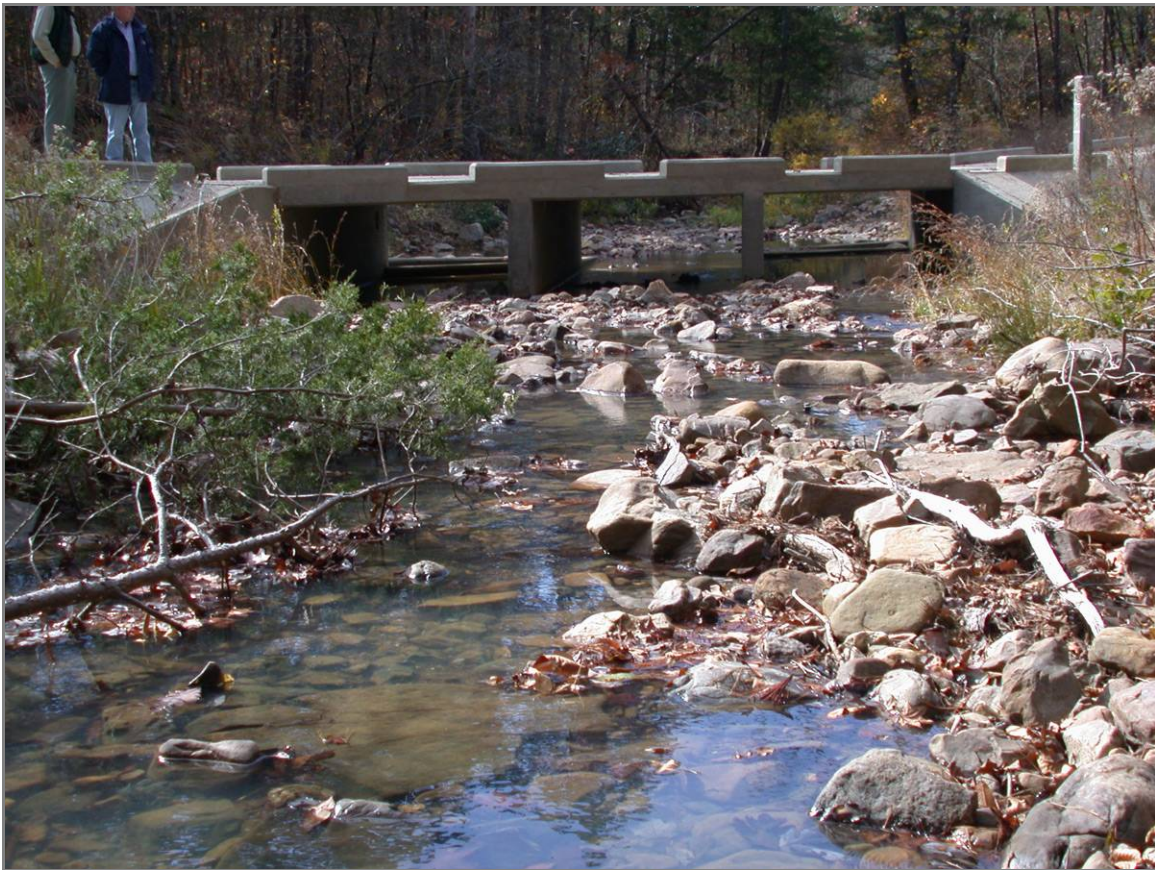
Figure 6 – Example of a Vented Ford type low-water crossing on the Ouachita National Forest, Arkansas. From the FishXing Case Studies website ( http://www.stream.fs.fed.us/fishxing/ ).
