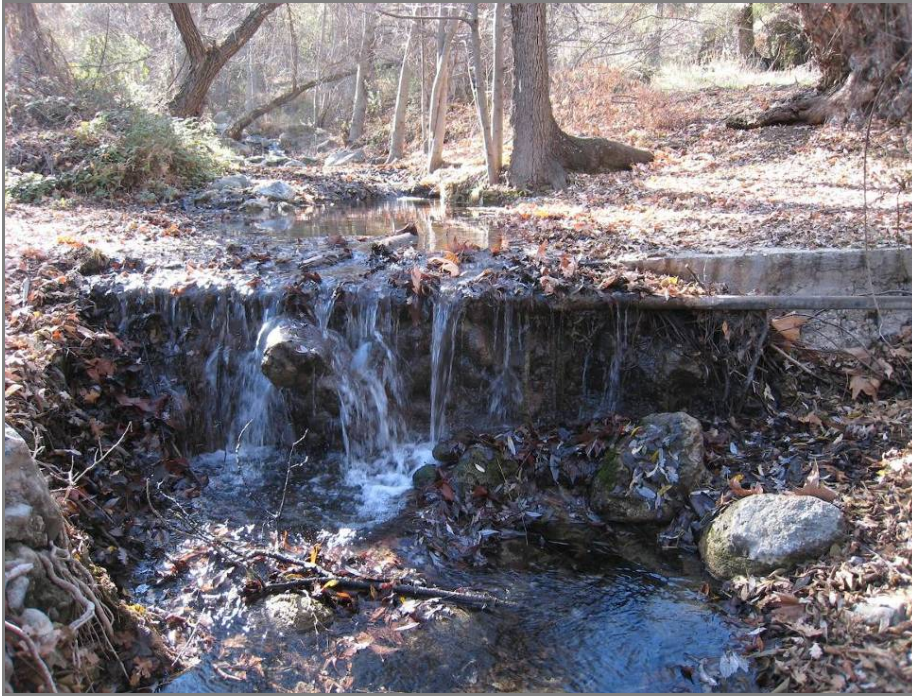
Figure 25 –Munch Creek crossing (H-150'59-1) is an abandoned 13-foot wide concrete low-water ford. Complete removal is recommended.
