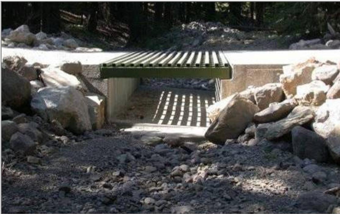
Figure 23 – Example of modifying an existing low-water crossing by cutting and forming a new box to create a vented ford. The crossing is designed using hydraulic criteria for fish passage and will not retain a natural streambed. The grate is removable to clear debris that may accumulate during high flows.
