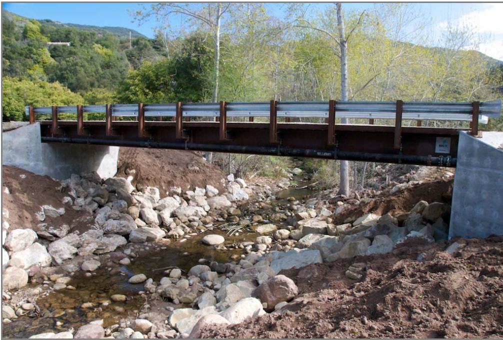
Figure 7 – Completed bridge installation for fish passage on Carpinteria Creek 2009.
