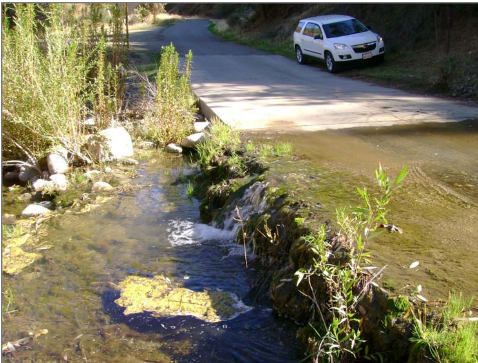
Figure 9 – Drop at the downstream edge of the low-water crossing on the lower Sunset Valley Road crossing at Davy Brown Creek.
