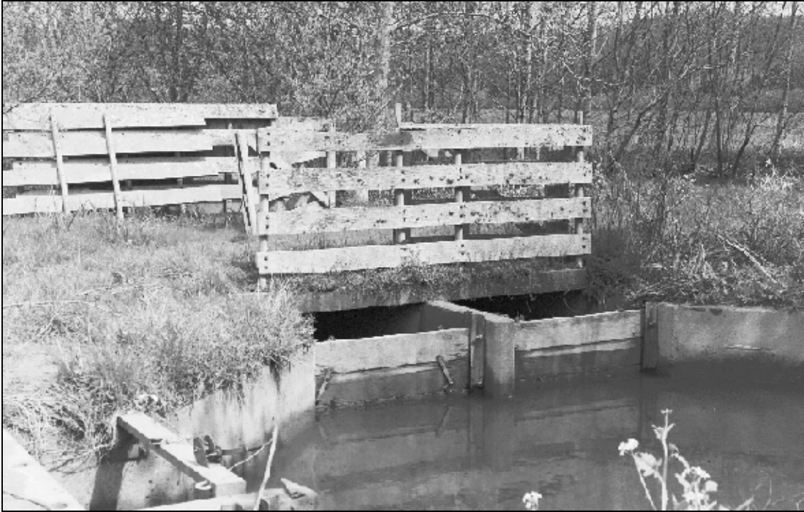
Figure 4.8 - The First Diversion located on Salmon Creek. Once water levels overtop flashboards flow is routed to other portions of the Refuge.
