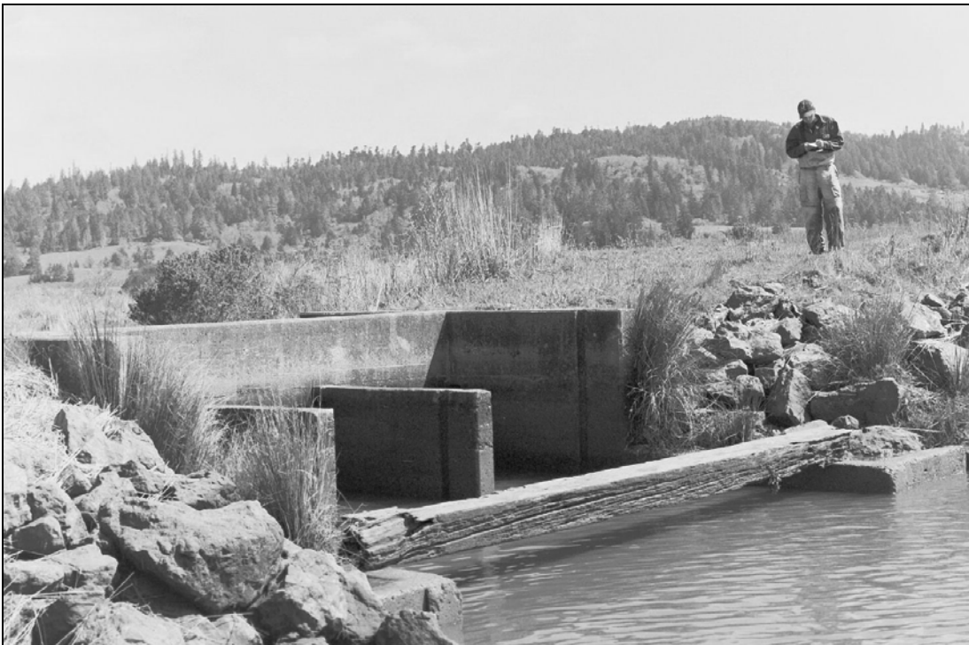
Figure 4.3 - Downstream side of Salmon Creek tidegate at Hookton Slough. Structure has three rectangular bays with top-hinged flaps. Far right bay contains a small opening to allow fish passage when flaps are closed.
