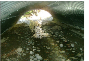
Woodacre Creek Stream Simulation Arch Culvert: Marin County, Michael Love & Associates, Stetson Engineers
