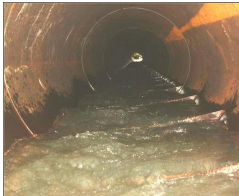
John Hatt Creek Slip-lined Culvert with Corner Baffles at High Passage Flow: CalTrans
