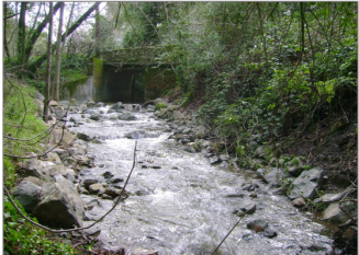
Woodacre Creek Roughened Channel Eliminates Culvert Outlet Drop: Marin County, Michael Love & Associates, Stetson Engineers
