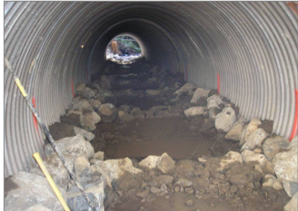
Gulch 7, Step-Pool Roughened Channel Culvert with Bed Retention Sills: Michael Love & Associates, Campbell Timber
