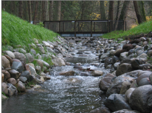
Spanaway Creek Bypass Chutes-and-Pools Roughened Channel Around a Water Supply Dam: Kozmo Bates
