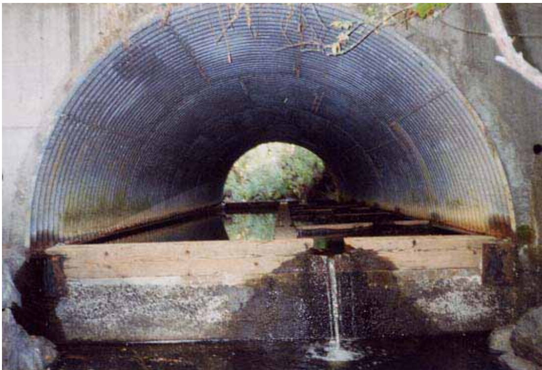
Cloney Gulch culvert outlet at summer low flow.
