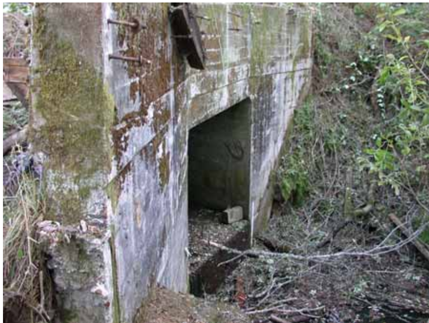
Upper McCready Gulch culvert outlet just prior to removal for replacement with a bridge.
