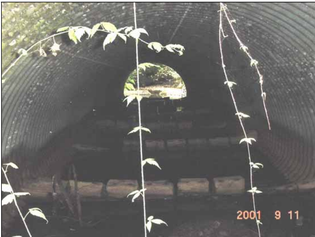
Peacock Creek North Bank Rd (Highway 197) culvert wooden baffles looking upstream.
