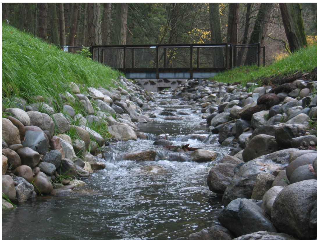
Figure XII-53. Spanaway Creek bypass roughened channel.
