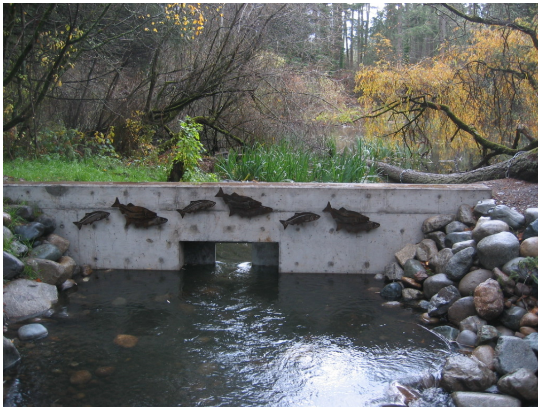
Figure XII-54. Flow control structure, Spanaway Creek bypass channel.
