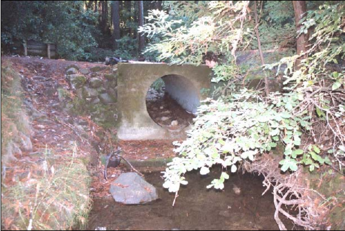
Culvert outlet and apron on McGarvey Gulch at the Richards Road-Trail crossing, Huddard Park.
