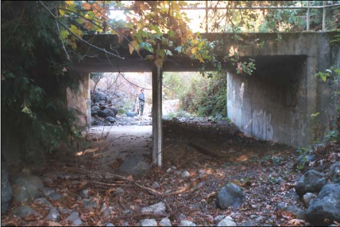
Inlet of the double bay box culvert at the Fire Access Road Crossing.
