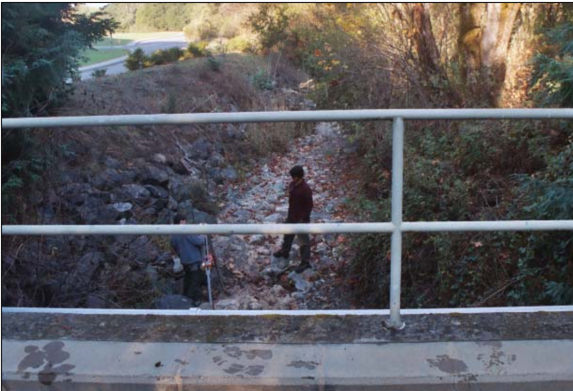
Channel bed downstream of the culvert outlet. Note the levee along the left bank that protects Valley Oak Road from flooding.
