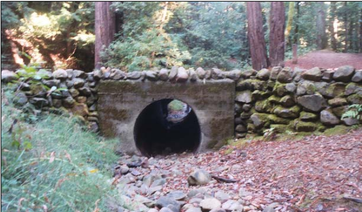
Culvert inlet on McGarvey Gulch. Note the added stone headwall and aggraded channel upstream of the inlet.
