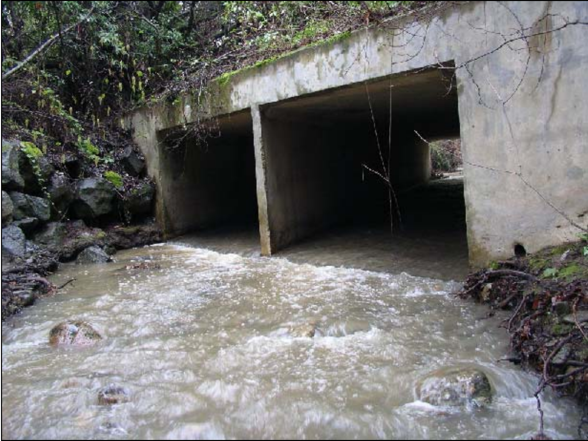
Los Trancos Creek double bay box culvert outlet on Los Trancos Creek (photo by Matt Stoecker)
