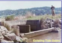
The existing 1.5'x3' fish door within the tidegates produces a "muted tidal cycle" inside the levees.
