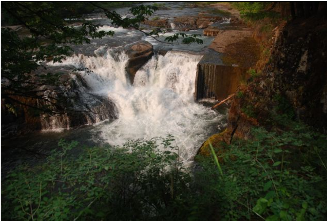
Photo 20. Estimated Flow of 151 cfs. Note flow beginning to overtop at both the upstream end and downstream end of the fishway roof. Nearly half the flow is bypassing the headwater pool as it goes over the falls.
