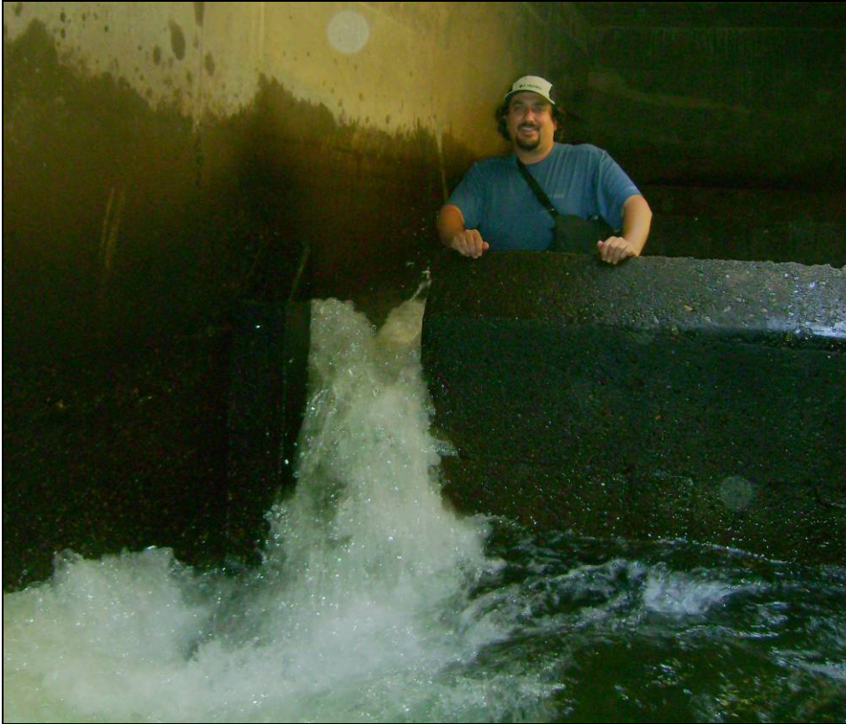
Photo 11. Slotted concrete weir with nearly 3-foot drop in the water surface due to large cobbles clogging the bottom of the slot.
