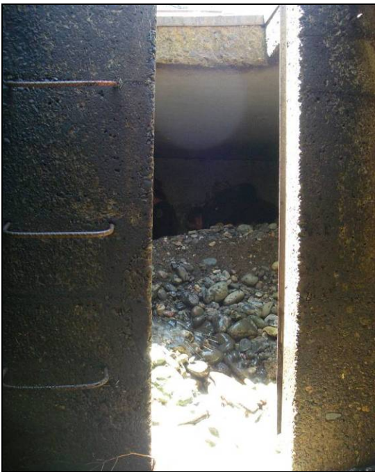
Photo 12. Sedimentation in the exit channel between the exit ports and Slot 20. Taken during annual cleanout on July 3, 2009. (photo courtesy of ODFW)
