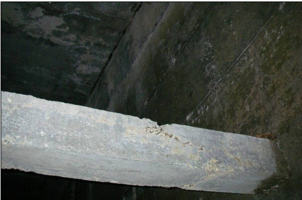
Photo 14. Spalled concrete on cross-member inside fishway (photo courtesy of ODFW).
