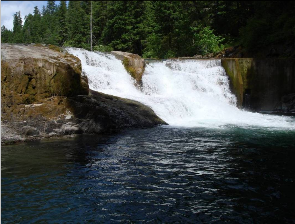
Photo 19. Estimated Flow of 123 cfs. Substantial proportion of streamflow bypassing spillway. No flow spilling off fishway roof.
