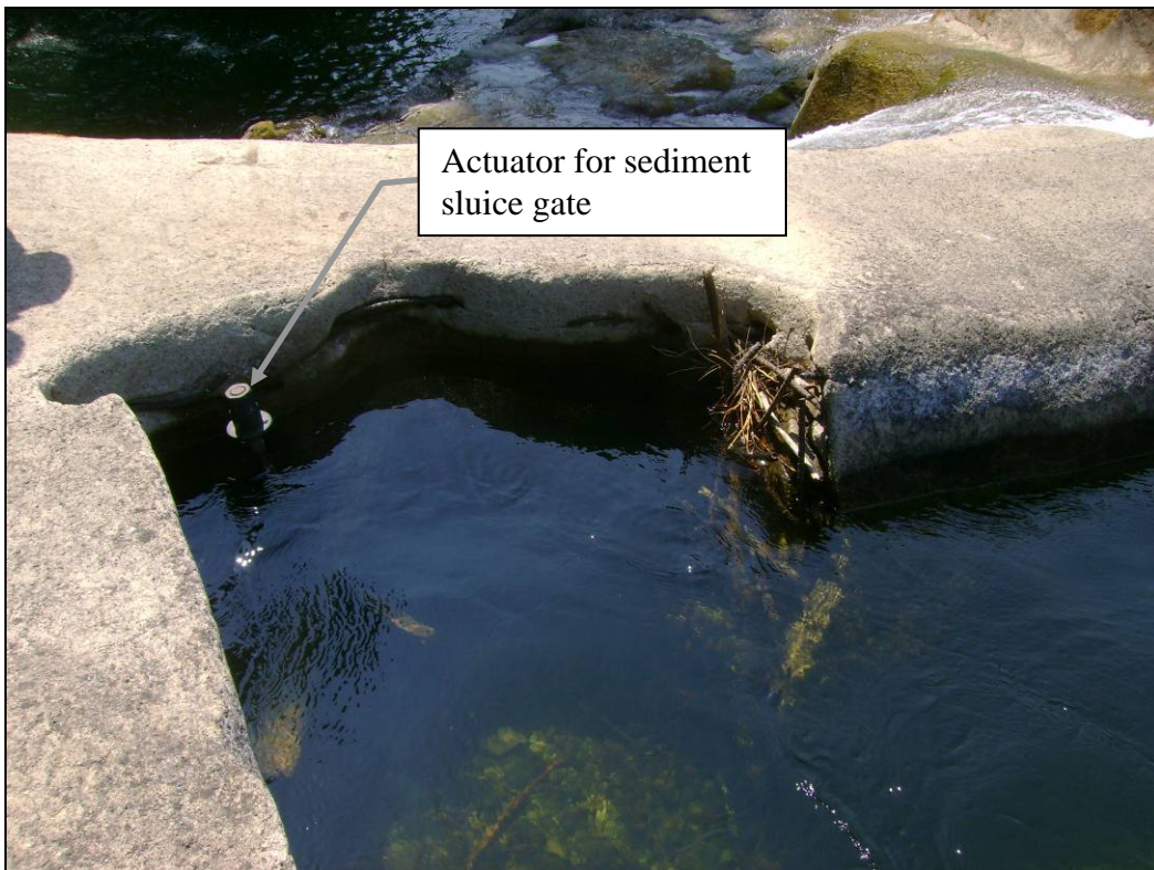
Photo 8. Damaged actuator for the sediment sluice gate on the spillway crest.
