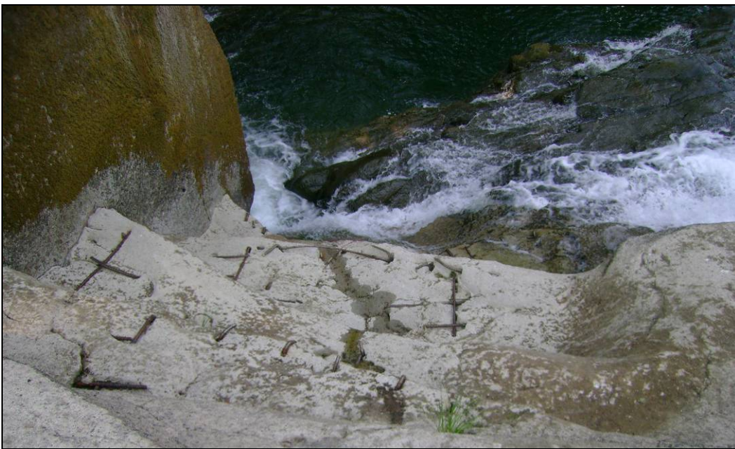
Photo 16. Rebar exposed on face of concrete spillway.
