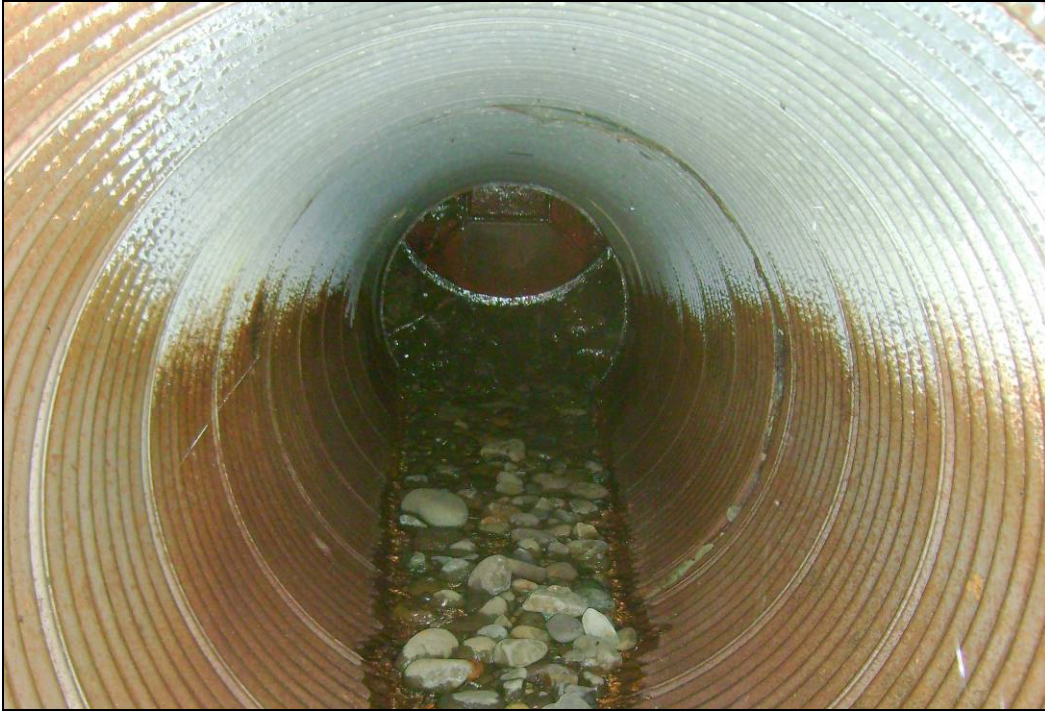
Photo 7. Looking up the sediment sluice pipe at partially opened slide gate plugged with sediment.
