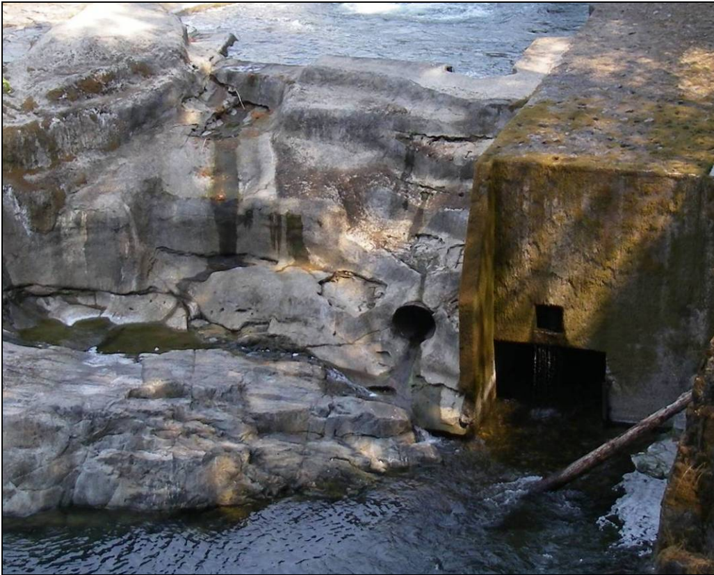
Photo 15. Concrete spillway and fishway exit at low flows, with all streamflow conveyed in fishway. Note spalled concrete and rebar exposed in numerous locations on the face of spillway.
