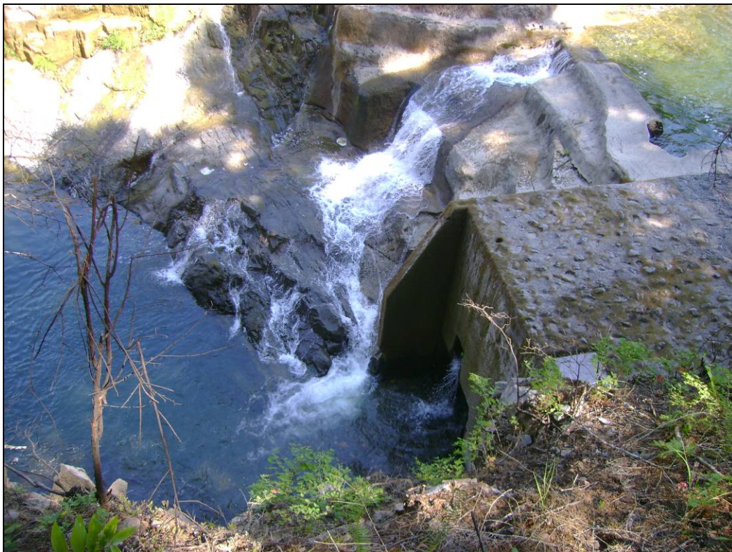
Photo 4. Looking down from the adjacent campground to the fishway entrance. At low flows the water going over the spillway is directed towards the entrance, which is likely beneficial for attraction.
