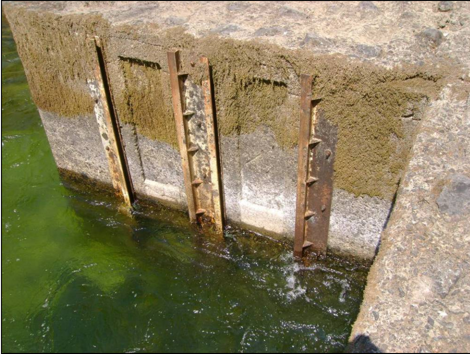
Photo 9. Exit ports (underwater) and stoplog guides in headwater pool.
