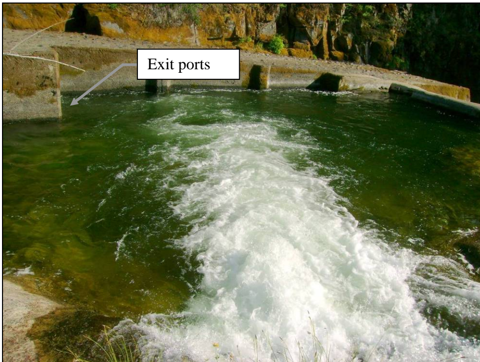
Photo 10. Flow entering the headwater pool scours the face of the exit ports, preventing sediment buildup.
