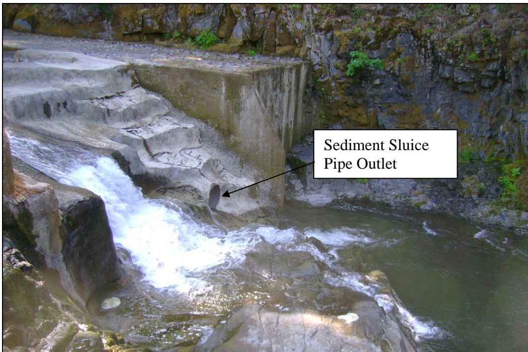
Photo 6. Fishway entrance and spillway. Note the outfall of the sediment sluice pipe for the headwater pool.
