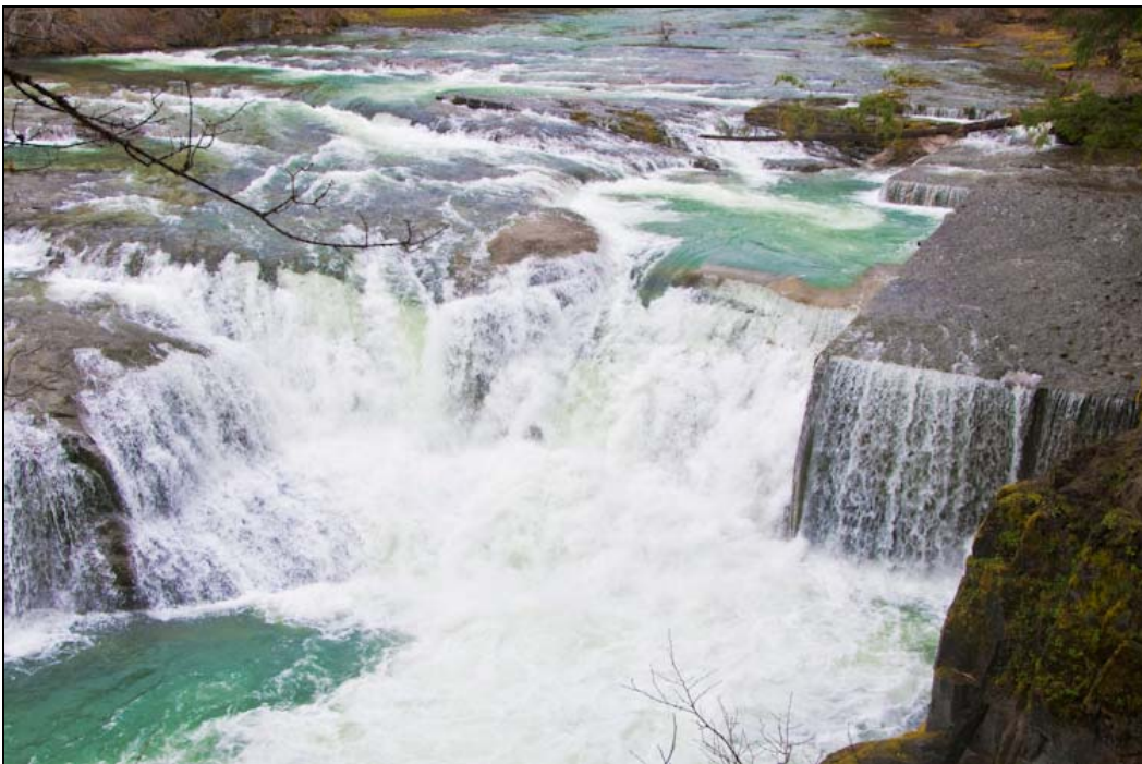
Photo 24. Estimated Flow of 519 cfs. Note the turbulence at the fishway entrance.
