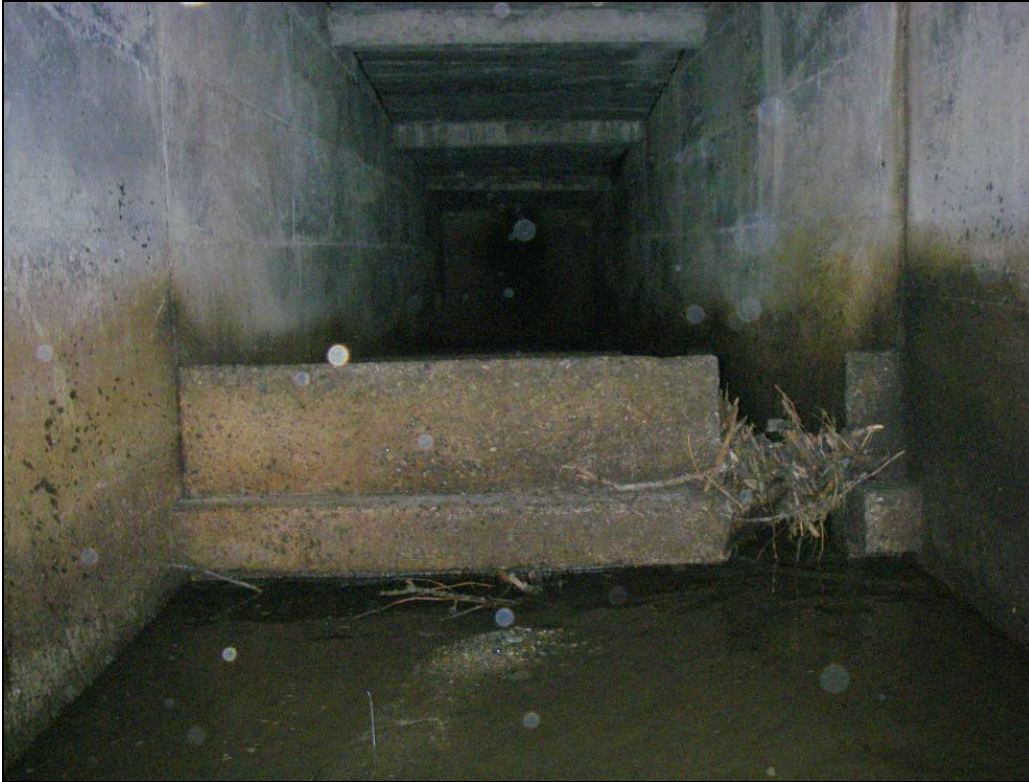
Photo 13. Small woody debris clogging Slotted Weir 18, taken during annual cleanout on July 3, 2009. (photo courtesy of ODFW).
