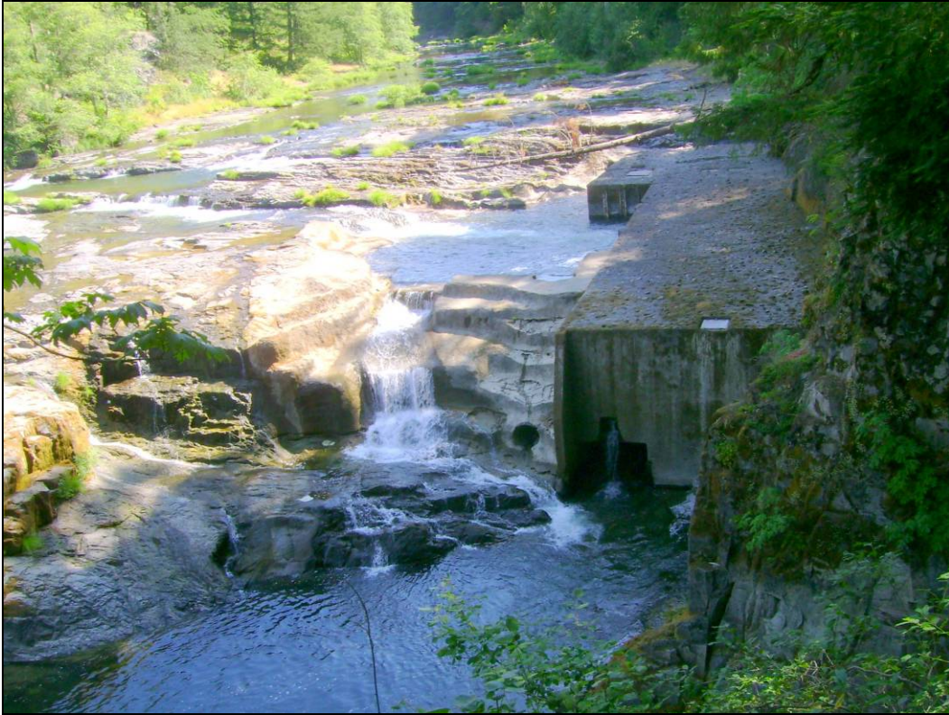
Photo 1. Looking upstream at the Steamboat Falls, the concrete spillway and headwater pool, and the fishway exit.
